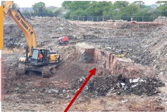
clay stank dividing the waste cells
